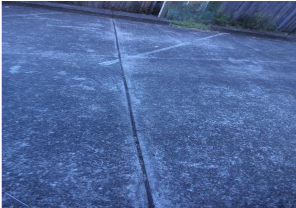
Photo 7 - 117-119 External, presumed asbestos bituminous expansion joints to concrete slab.
