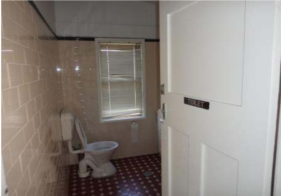
Photo 17 - 125, Internal, Level 1, presumed asbestos cement wall & ceiling linings in bathroom.
