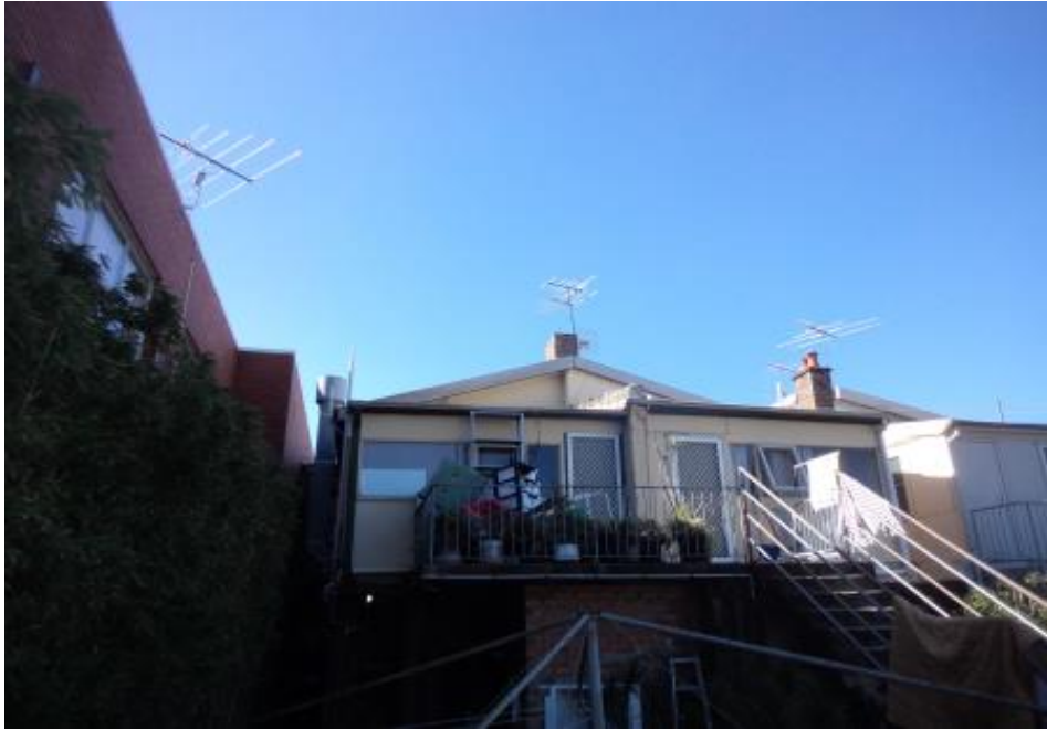
Photo 11 - Units 1 & 2, presumed asbestos cladding and gable end to roof.
