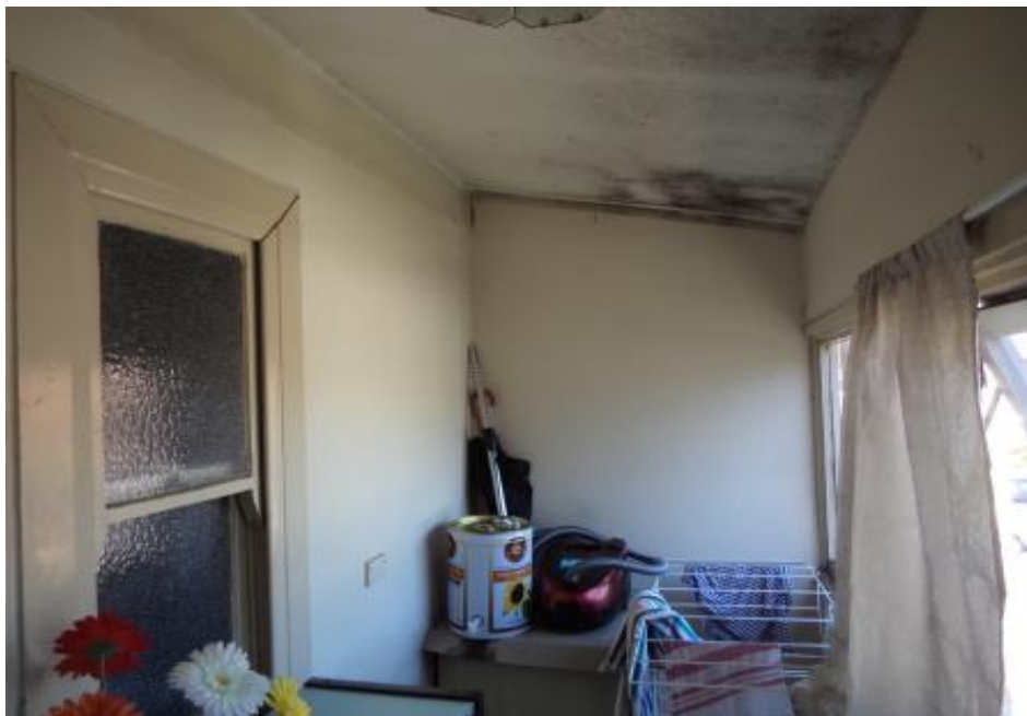
Photo 12 - Unit 2, presumed asbestos cement ceiling and wall linings.
