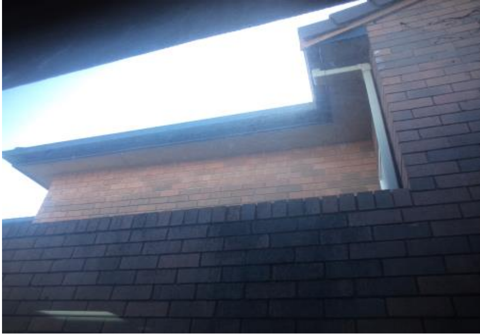
Photo 1 - 111, External, presumed asbestos-containing cement eaves.
