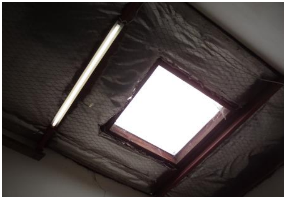
Photo 20 - 117-119, SMF sarking to roof.
