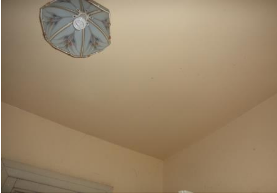
Photo 13 - Unit 2, presumed asbestos cement ceiling and wall linings.
